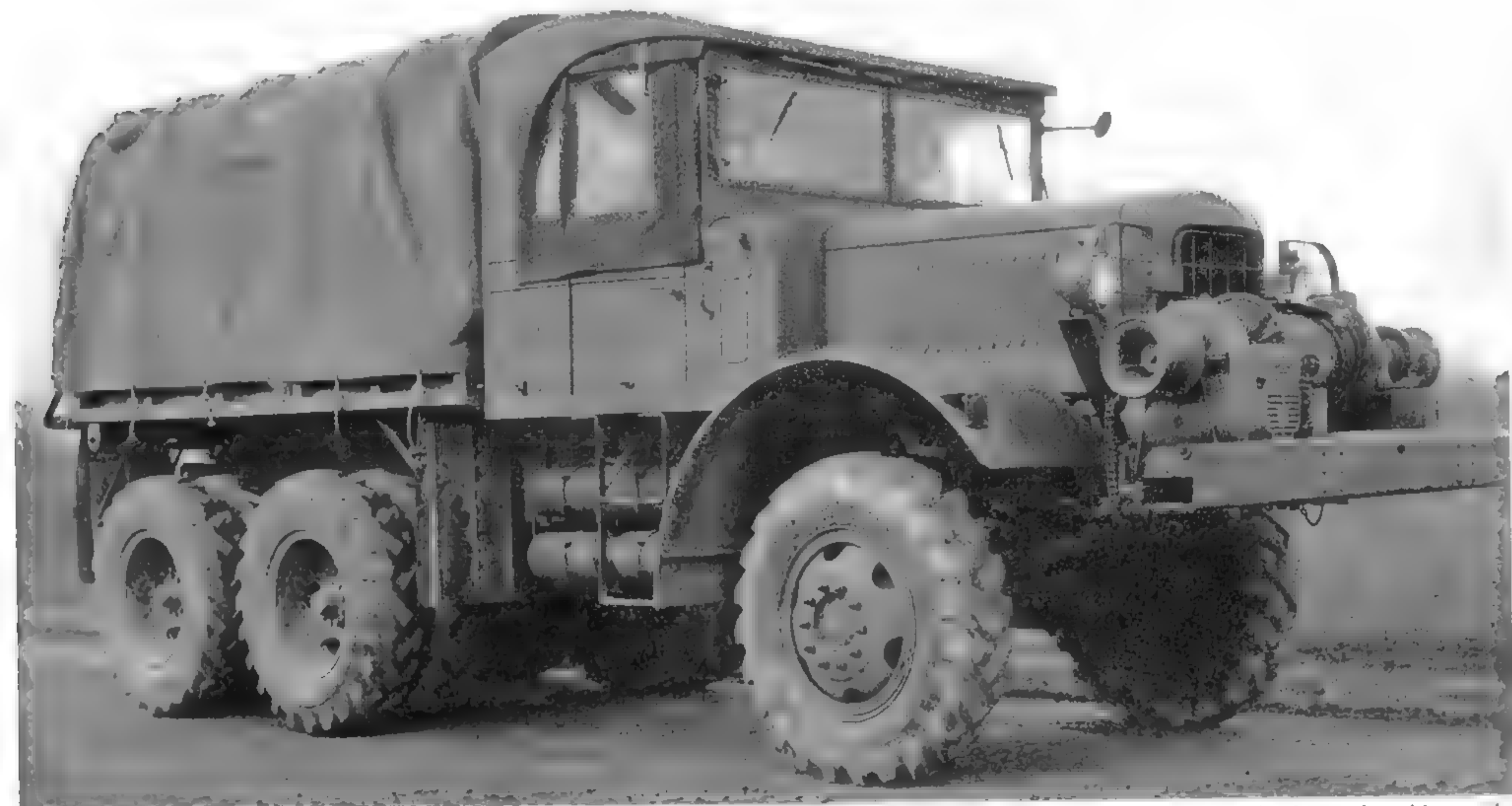
The lone Mack model NO was photographed at Aberdeen Proving Ground in December of 1940. Unlike the production models, the engine side panels of this truck were louvered, and the cab was the traditional Mack C shape. Even with the antique-style cab, the NO was an impressive machine, and the huge winch behind the front bumper did nothing to diminish its brawny look. (National Archives and Records Administration photo)
